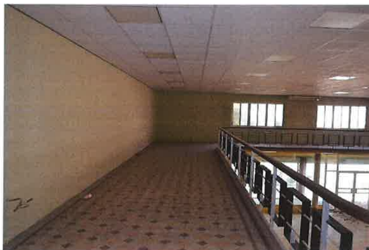
Inside of the building
