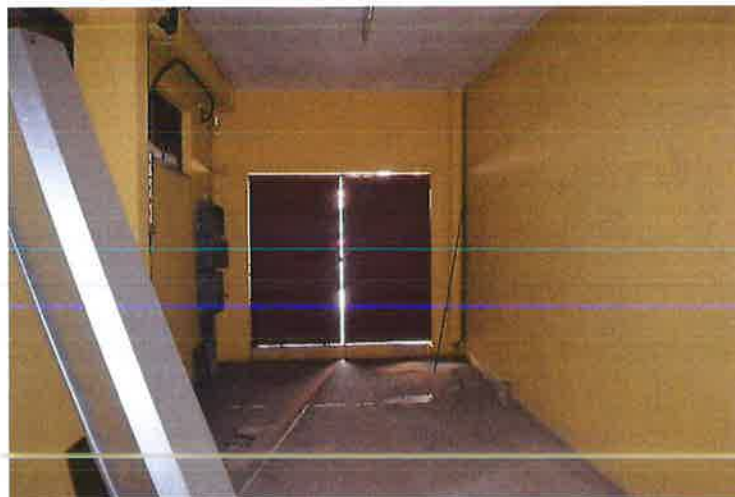
Inside of the building
