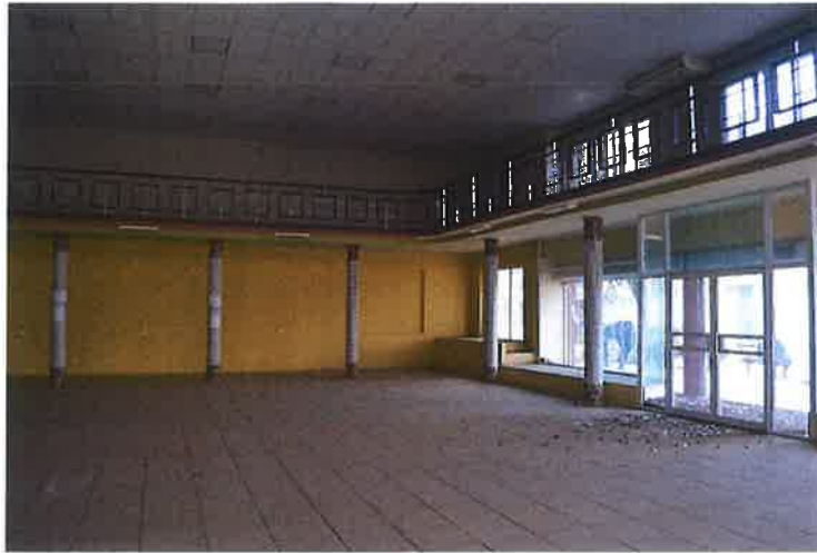
Inside of the building
