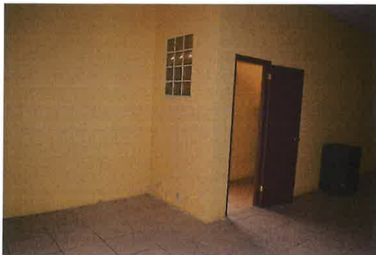
Inside of the building
