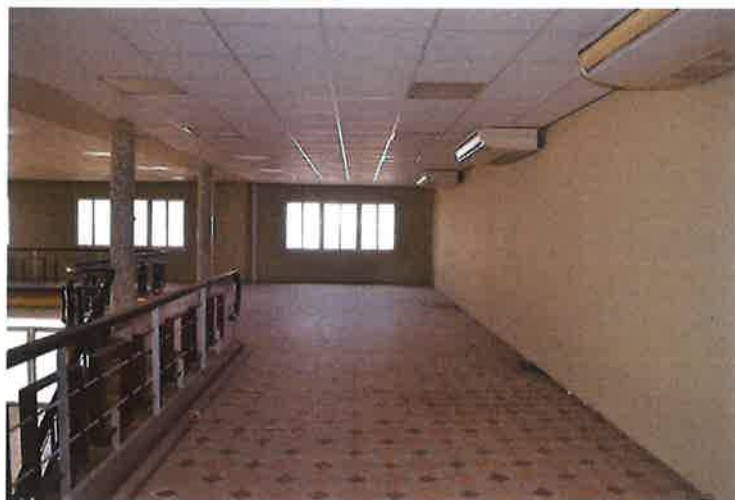
Inside of the building
