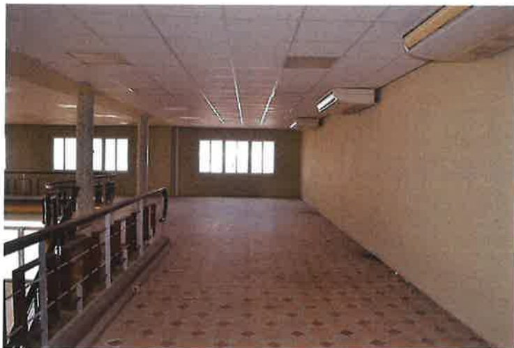
Inside of the building
