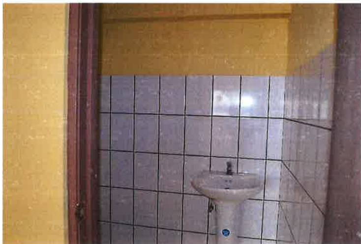
Inside of the building
