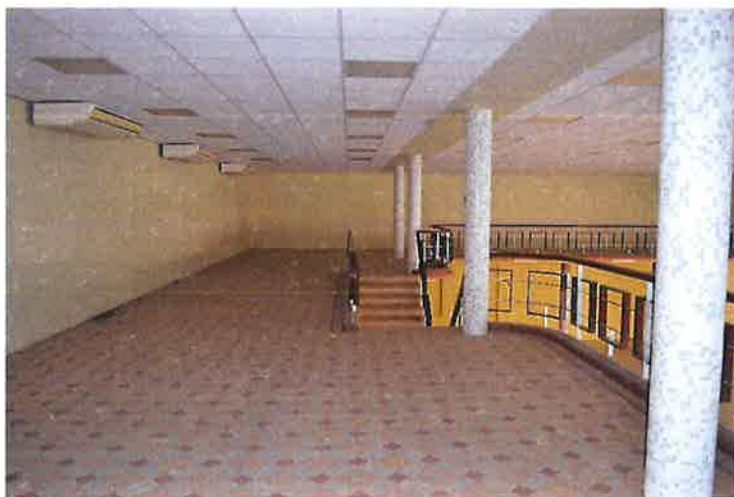
Inside of the building
