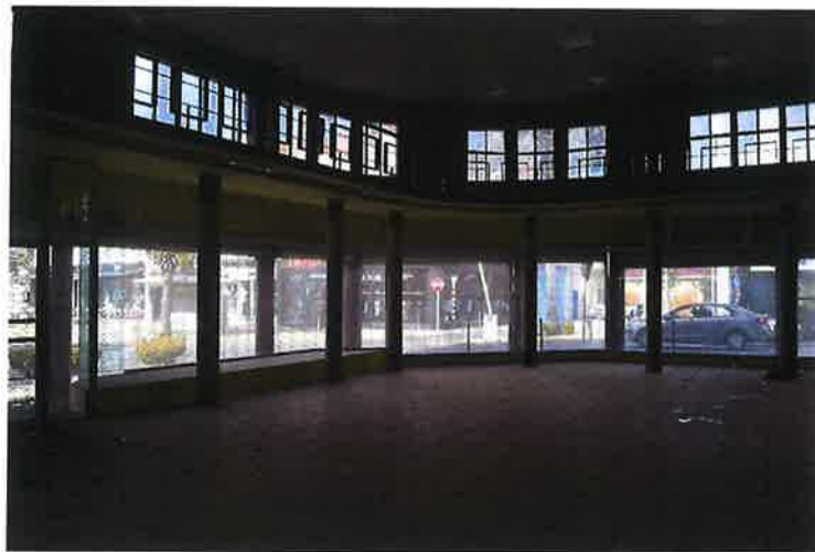
Inside of the building
