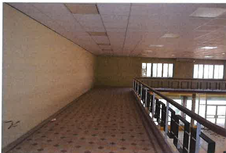
Inside of the building
