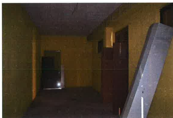
Inside of the building
