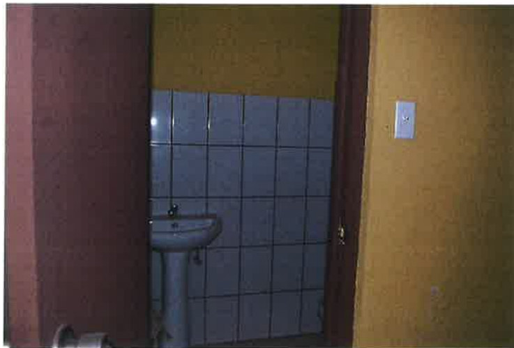
Inside of the building
