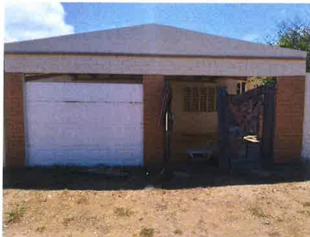
Left Façade / Entrance to Garage
